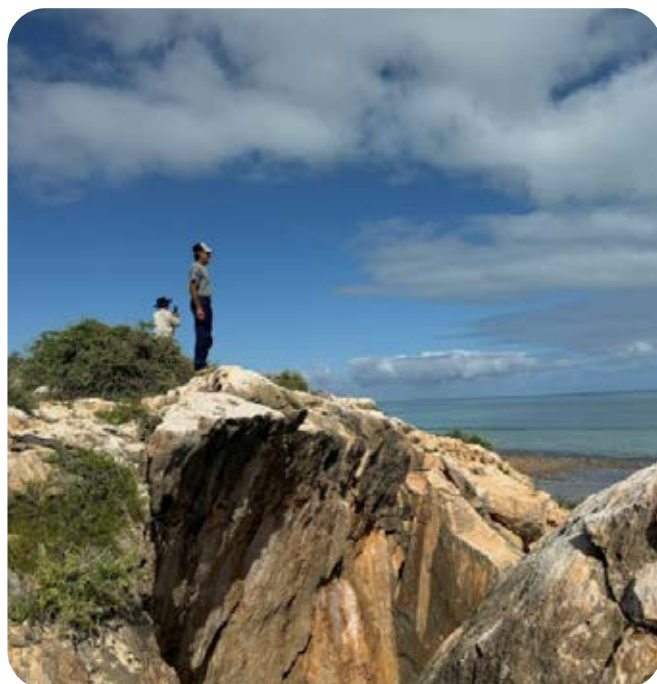
Inspecting the erosion site at Flint Cliffs (image: Cameron Perrett).
