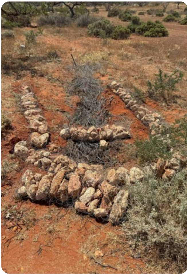
Malgana Rangers built locally sourced 'rock sieves' to help control erosion (image: Cameron Perrett).
