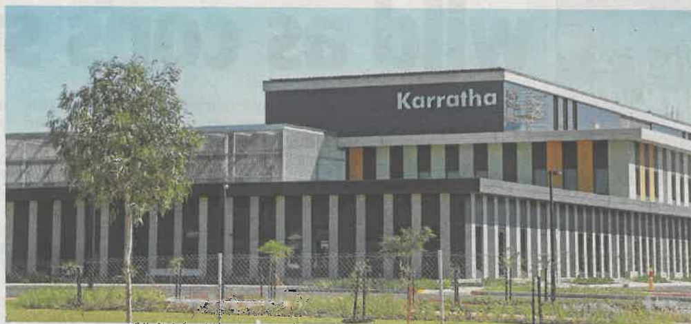
The $207.15 million Karratha Health Campus has reached practical completion. Picture: Alicia Perera
